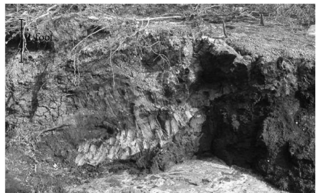
Fig. 5. View of the exit of the upper failure surface (Toe Scarp No.1), at the inboard toe of the laterally translated embankment (IPET 2006)
