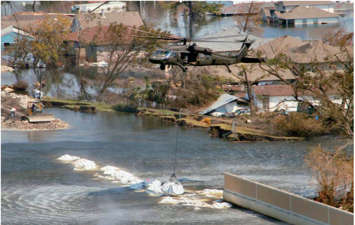
Fig. 2. (Color) Breach at the East Bank of the 17th Street Drainage Canal (USACE 1990)
